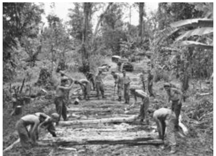
1945 Bougainville Island. Pioneers of the 9th infantry battalion building a corduroy road through the jungle Source: Australian War Memorial
